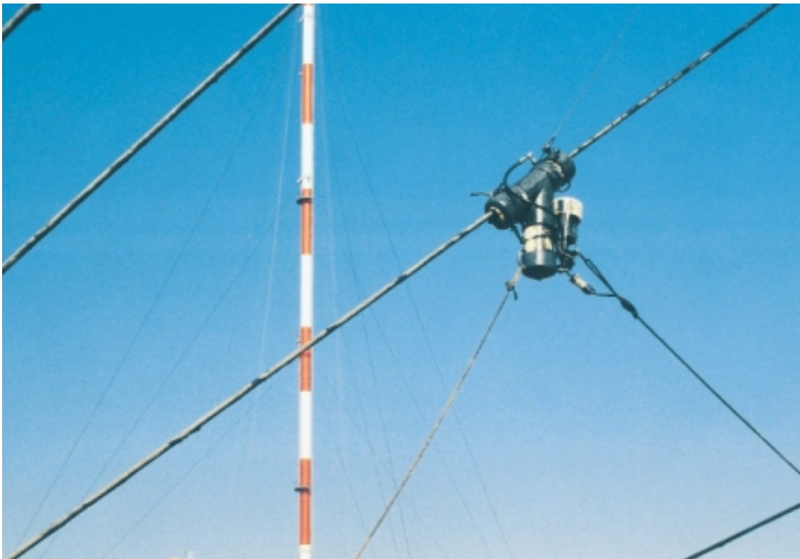
Lubricating tool applying synthetic penetrating lubricant
